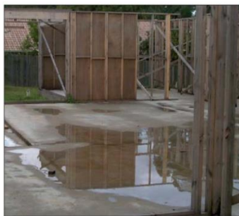
The puddles indicate low areas in this slab
