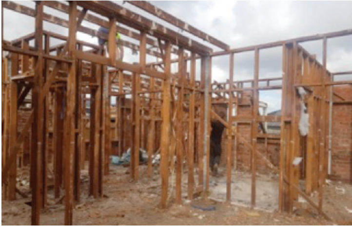
Hand remove the timber from the demolition site.
